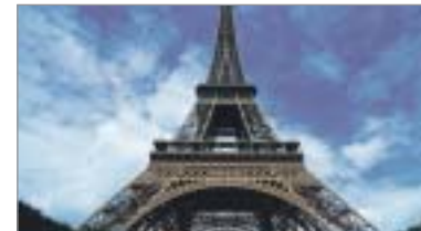
For safe ascent and descent: KABELSCHLEPP cable carriers in the Eiffel Tower, Paris.
